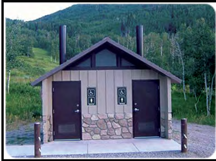
Figure 4-7. Vault Toilet Example.
