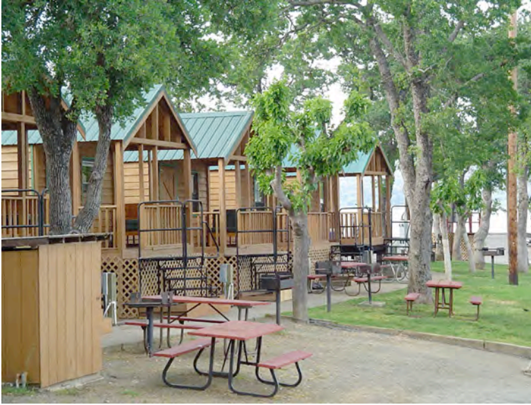
Lake Berryessa Marina Resort - Cabin / Modular Units
